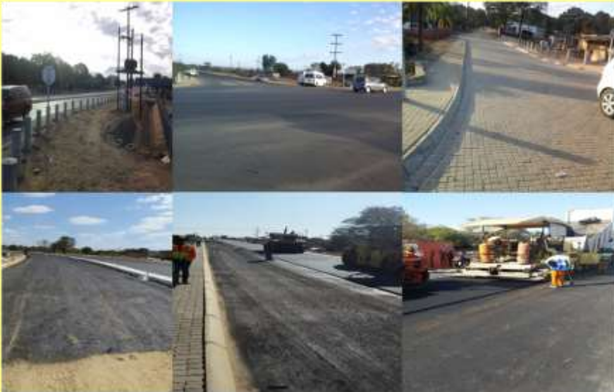
Section A upgrading from gravel to tar
