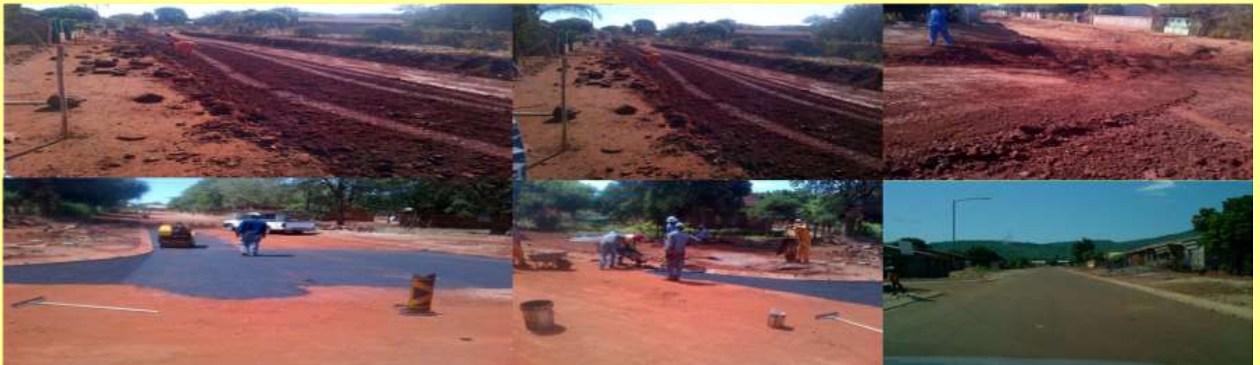
Section A upgrading from gravel to tar
